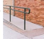
four-degree angle of rise are difficult to visually detect and may not be apparent to users, resulting in frequent tripping. Ramps are usually designed with rise angles between four and 15 degrees. Most building codes specify a slope of no greater than one unit vertical and eight units horizontal.
